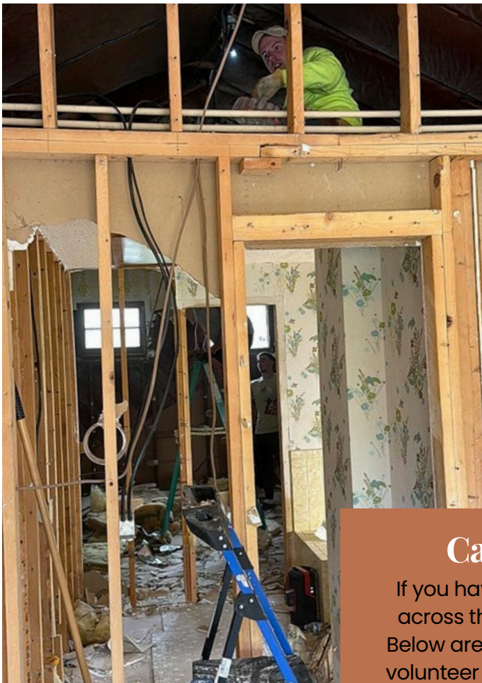
New Safe House Under Construction
